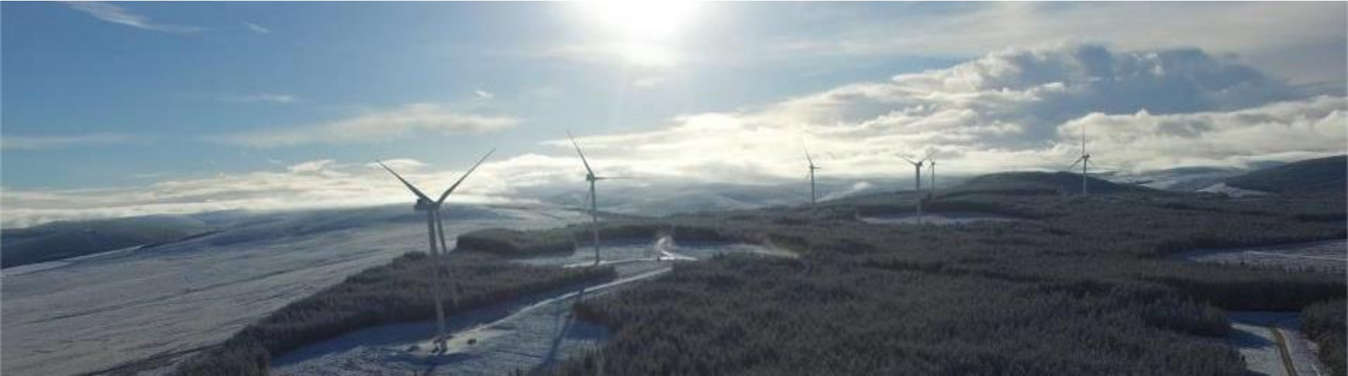
Andershaw wind farm, Scotland
